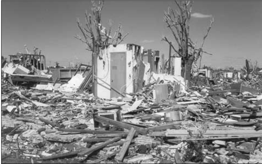
Figure 1-1 Small interior room that survived a tornado.
